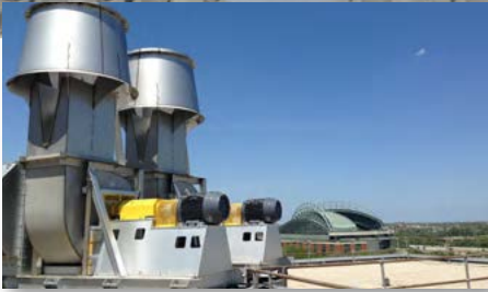
Model BCIFE Generator Exhaust
