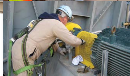
Coupling & Sheave Alignment
