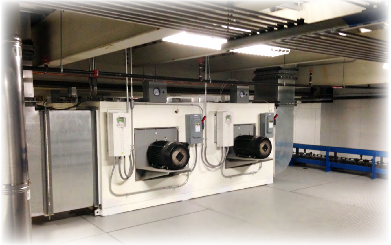
Recirculation Fans in Paint Finishing System
