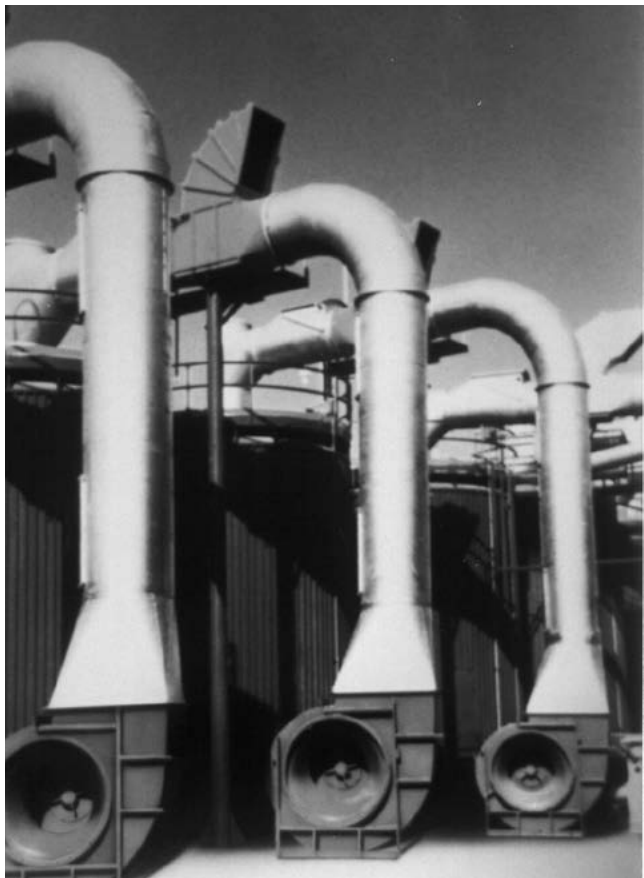
Figure 6. Well-designed duct configuration
